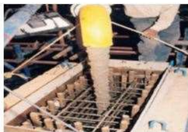
Fig. 3 Pouring of SCC by pumping
