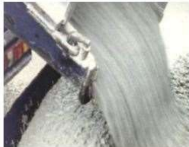
Fig. 1 Flow of SCC
