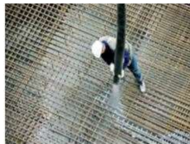
Fig. 2 Pouring of SCC in congested reinforcement
